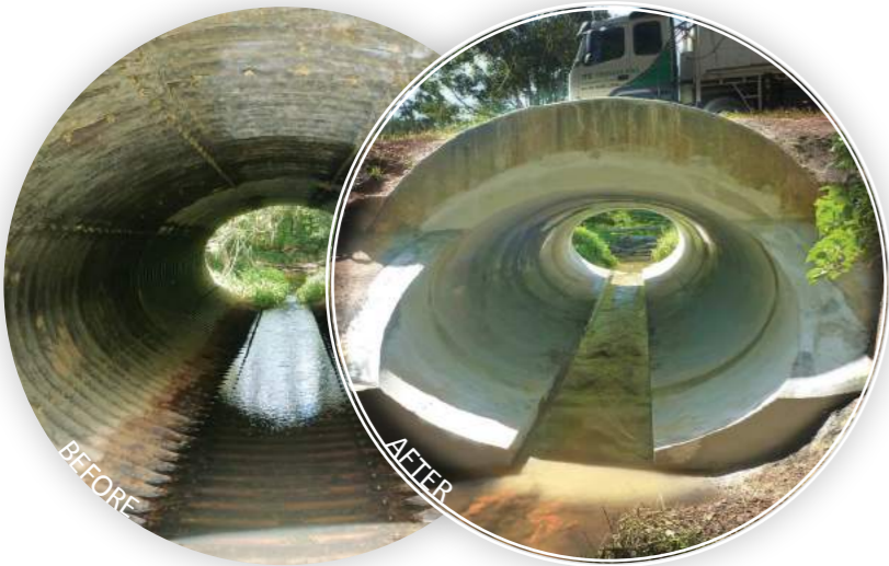
3700 x 2400mm Elliptical Corrugated Steel Culvert Location Burringbar, NSW Client Tweed Shire Council
